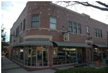
Façade, Awnings, and Signage (Wheaton) – Page 10
